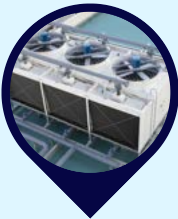
CROSSFLOW COOLING TOWER
